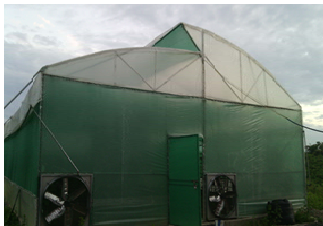
Fig. 1: High-tech poly green house structure
